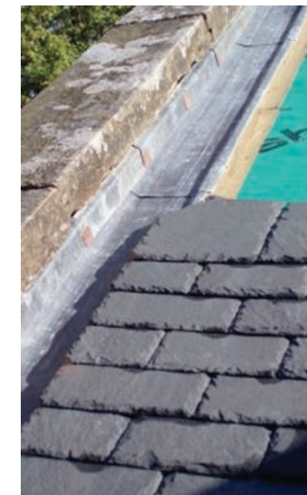
PRECEDENT PHOTO Typical secret gutter verge detail
