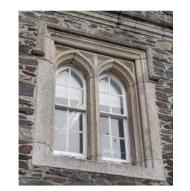
Subframe/ surround: To all granite mullions and window surrounds, strip back all paintwork Ironmongery: to be refurbished and/ or replaced where required. Finish: Paint windows with 2no. undercoats and finish with 1no. gloss finishing coat Colour: White - TBC External M60/123 Internal M60/150 Spec Reference: L10/210 Comments - Option A: No Draught Seals - Option B: Draught Seal weatherstrip around perimeter of sashes / recessed brush seal to sash meeting rail.
