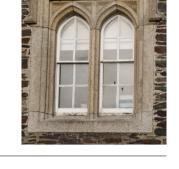
Subframe/ surround: To all granite mullions and window surrounds, strip back all paintwork. Ironmongery: to be refurbished and/ or replaced where required. Finish: Paint windows with 2no. undercoats and finish with 1no. gloss finishing coat Colour: White - TBC External M60/123 Internal M60/150 Spec Reference: L10/**210** Comments - Option A: No Draught Seals - Option B: Draught Seal weatherstrip around perimeter of sashes / recessed brush seal to sash meeting rail
