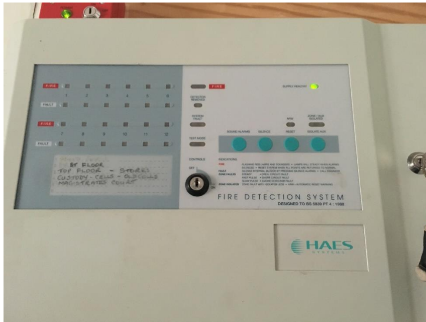
Photo 32.2.1: Existing fire alarm panel at high level (above doorway) shall be stripped out and removed
