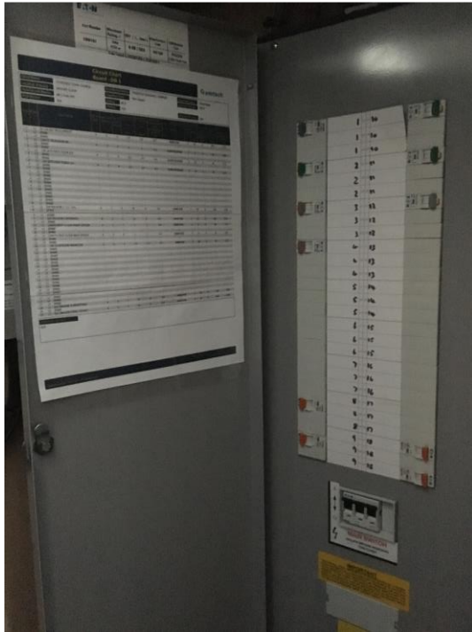
Photo 23.3.1: Recently up-graded panel board (shall be retained)
