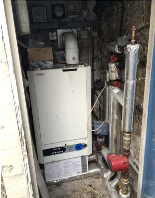
Photo 20.2.1: Existing boiler in lean-to boiler house (shall be stripped-out)
