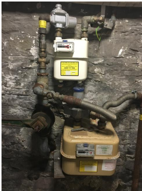
Photo 18.2.2: Existing gas meter(s) (U6 at H/L and U16 at L/L) located in one of the original cells
