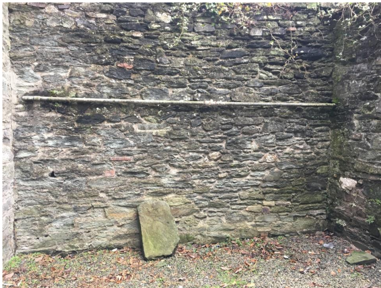
Photo 18.3.1: Surface mounted pipework (possibly gas) leaving the Guildhall (on the left) and heading towards the cottages (on the right). The Contractor shall survey and identify what this pip is before isolating and removing.
