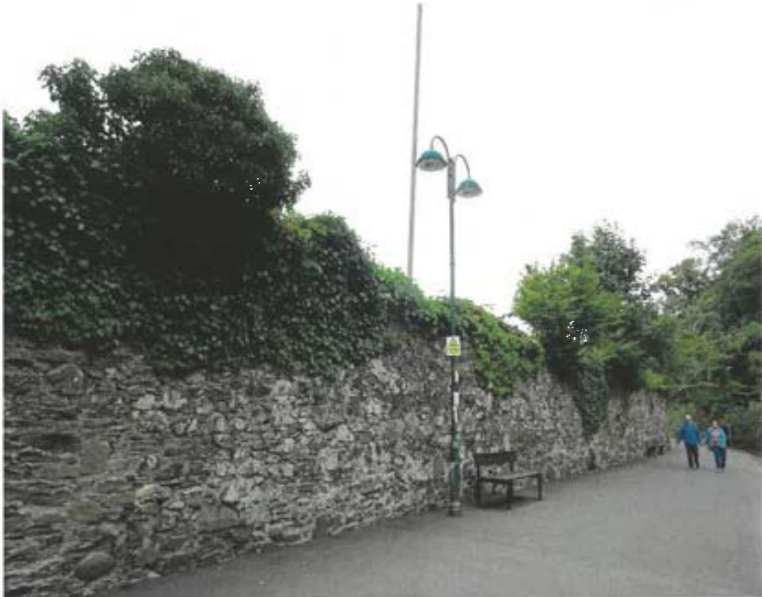
Wall looking east
