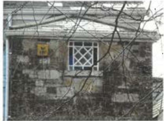
3 of 4 End porch window detail
