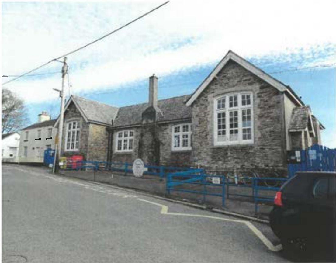
Former primary school from Church Hill
