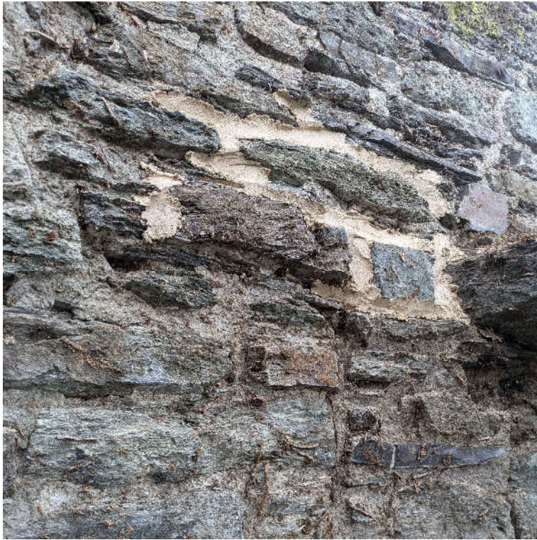
Image 19 – Internal face of north west elevation Root removed and section of stonework removed and rebedded in lime-based mix (unfinished pointing at time of photograph)
