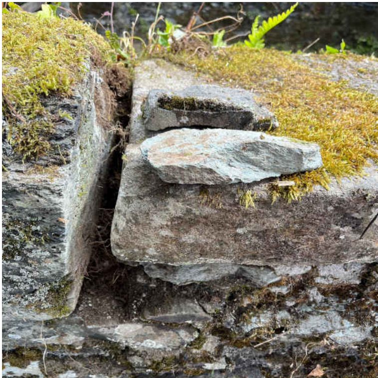
Image 16 – Top of wall to south west elevation Photo after root has been removed (prior to pointing)
