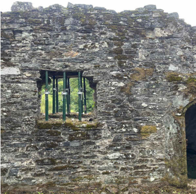
Image 06 – Internal view of south east elevation Props installed to window
