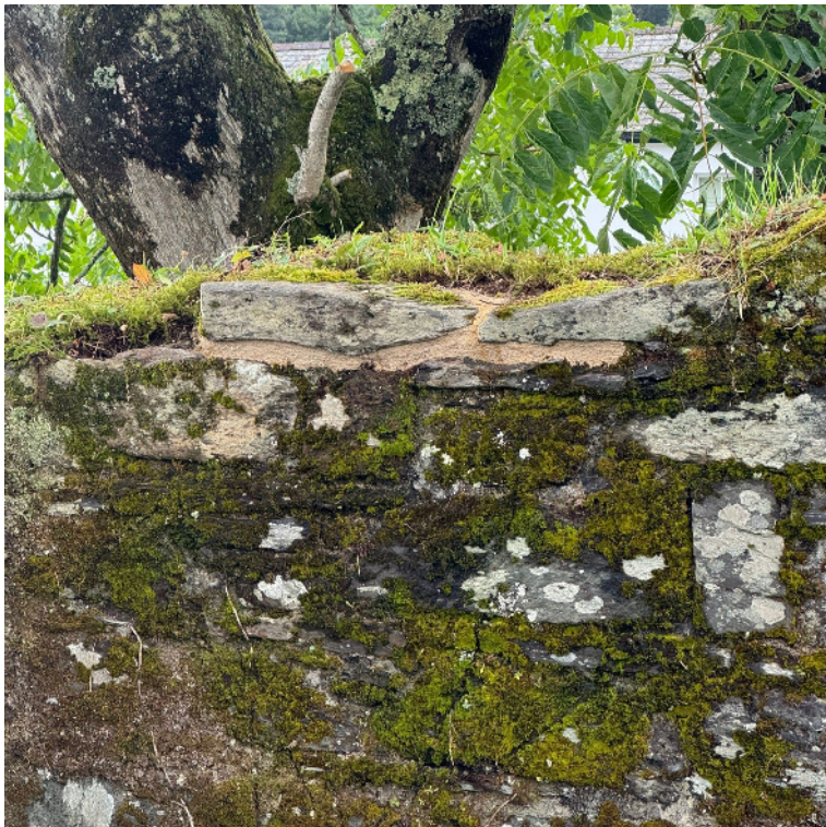
Image 18 – Top of wall to north west elevation Root removed and section of stonework removed and rebbed in lime-based mix
