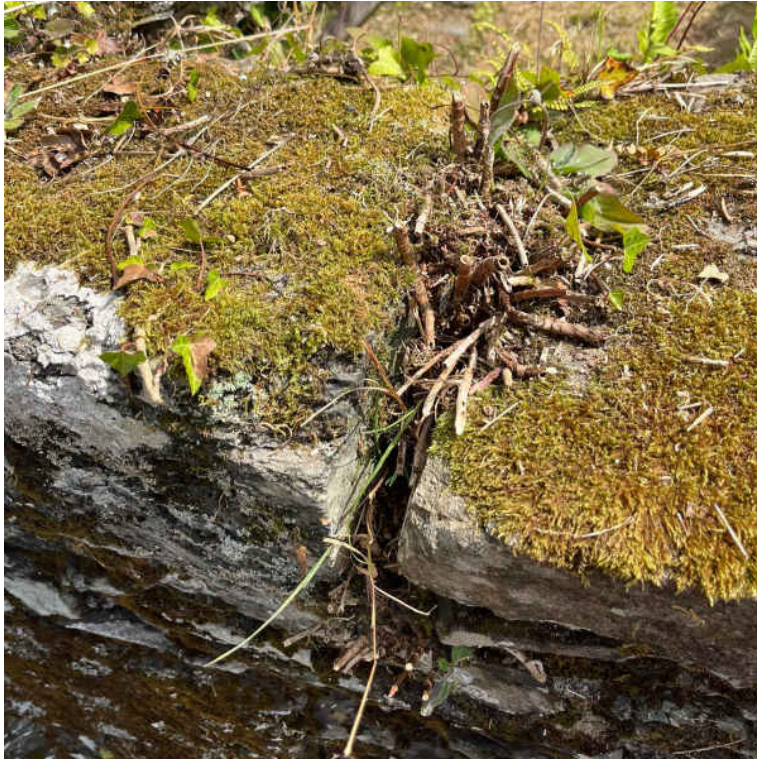
Image 15 – Top of wall to south west elevation Root to be removed
