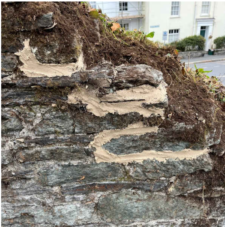
Image 20 – Top of wall to north west elevation Root removed and section of stonework removed and rebedded in lime-based mix (unfinished pointing at time of photograph)
