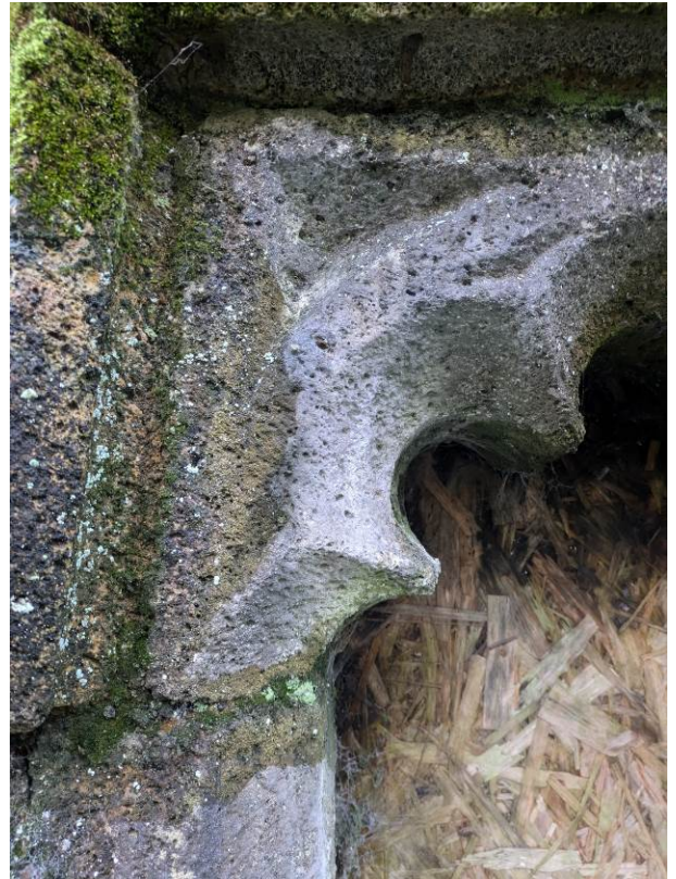
Erosion to Tracery on South Elevation Window ( Image 14 )
