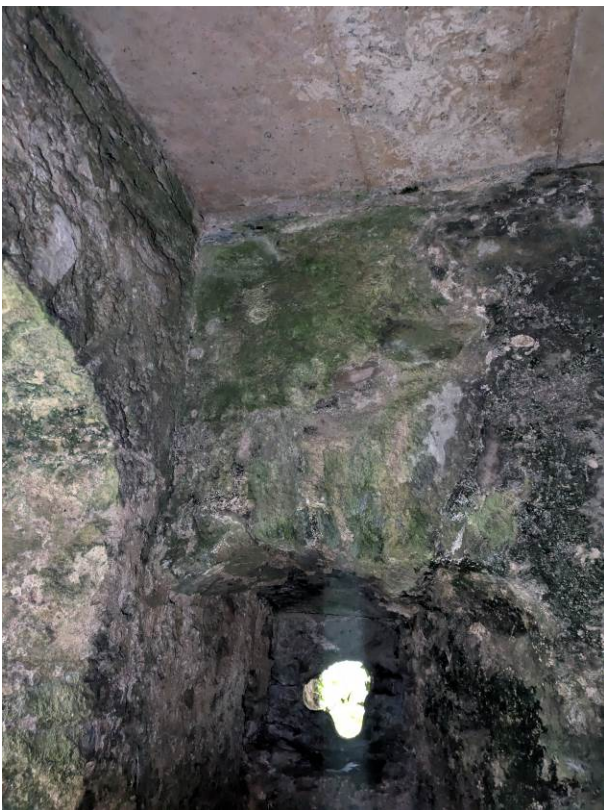
Ground Floor View of the North-West Corner Showing Signs of Biological Growth and Damp Stonework (Image 23)
