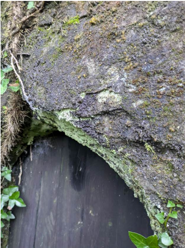
Tracery to Door on East Elevation Beginning to Erode ( Image 17 )
