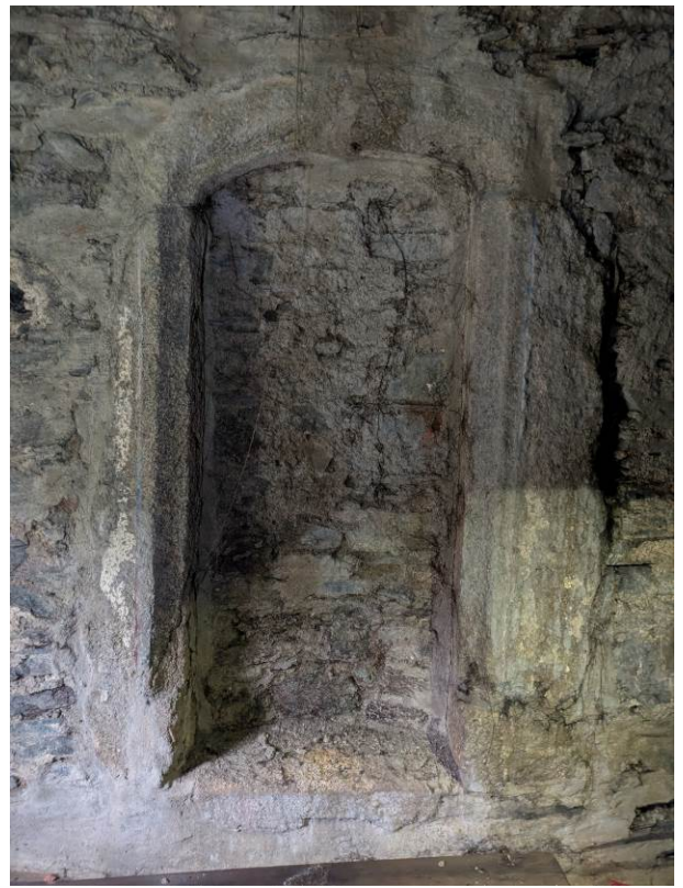
Blocked Door to East Elevation of Upper Level with Inappropriate Cement Slurry around it and Gaps in the Pointing (Image 22)
