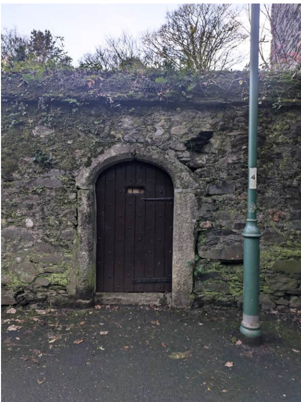
Gate to South Elevation with Sockets of Missing Stone to the Wall ( Image 11 )
