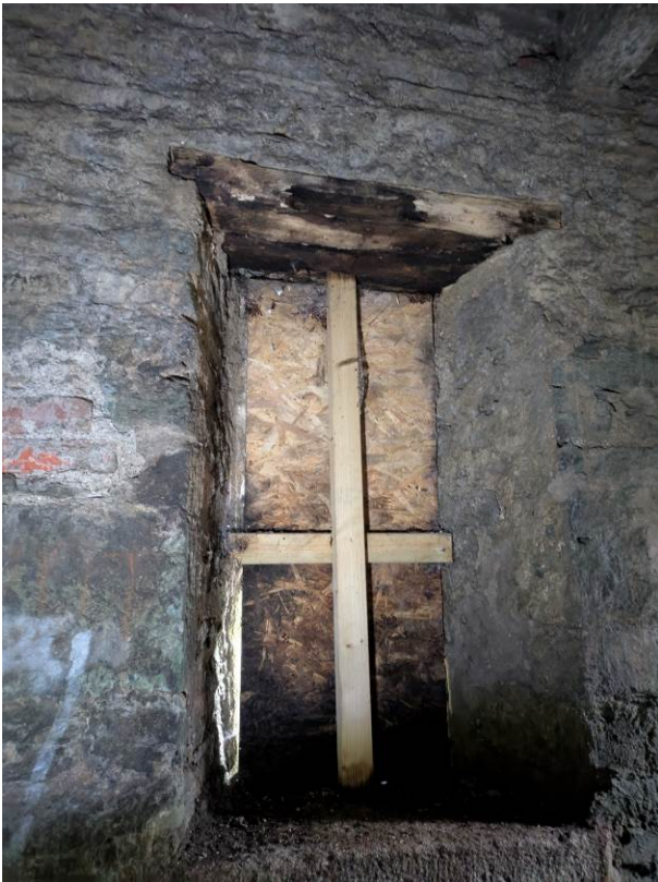
Rotten Timber Lintel to Window in West Elevation (Image 21)
