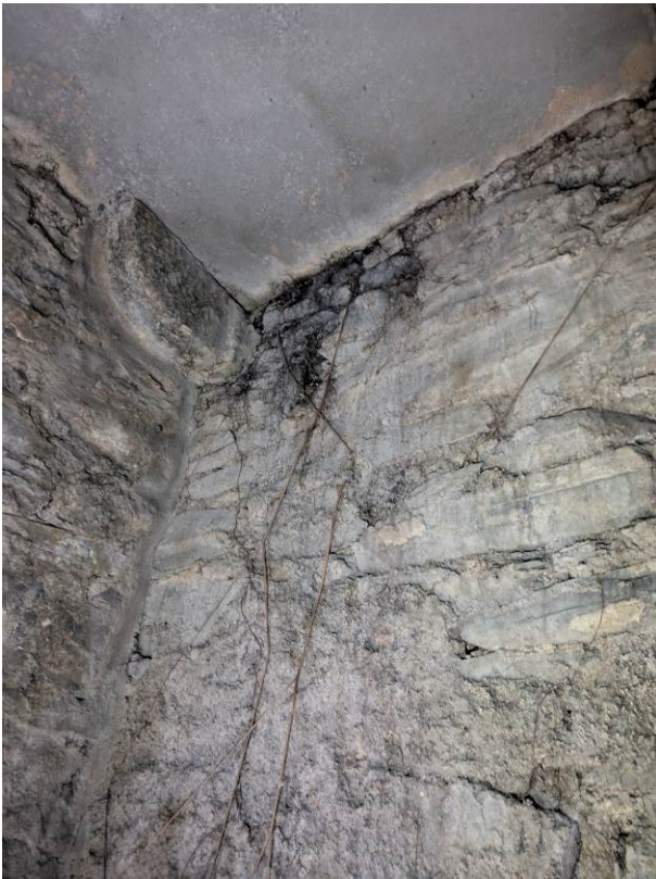
Roots coming into the east elevation and damp to high levels in the upper storey ( Image 25 )
