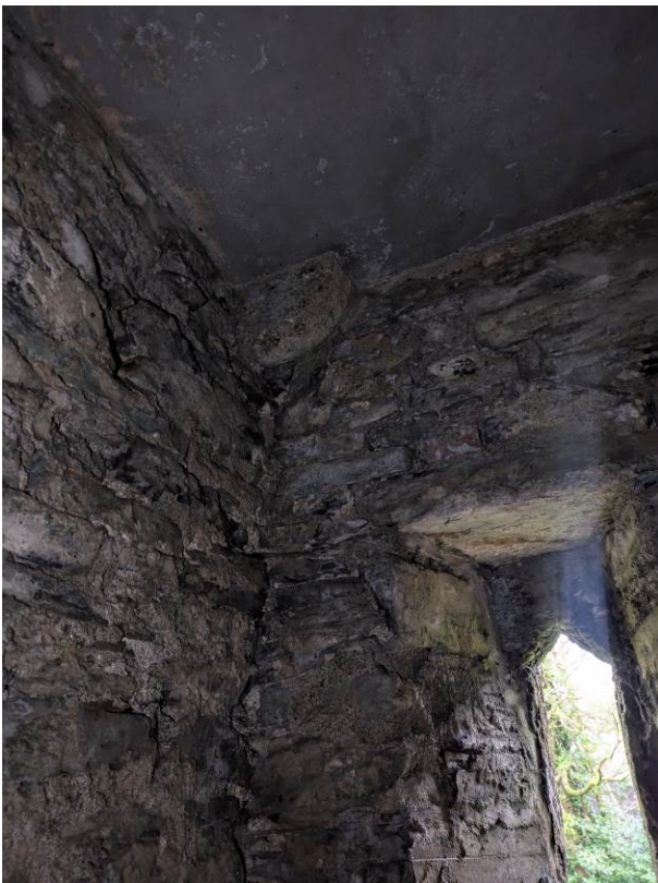
Upper storey north west corner showing missing pointing and evidence of damp ( Image 27 )
