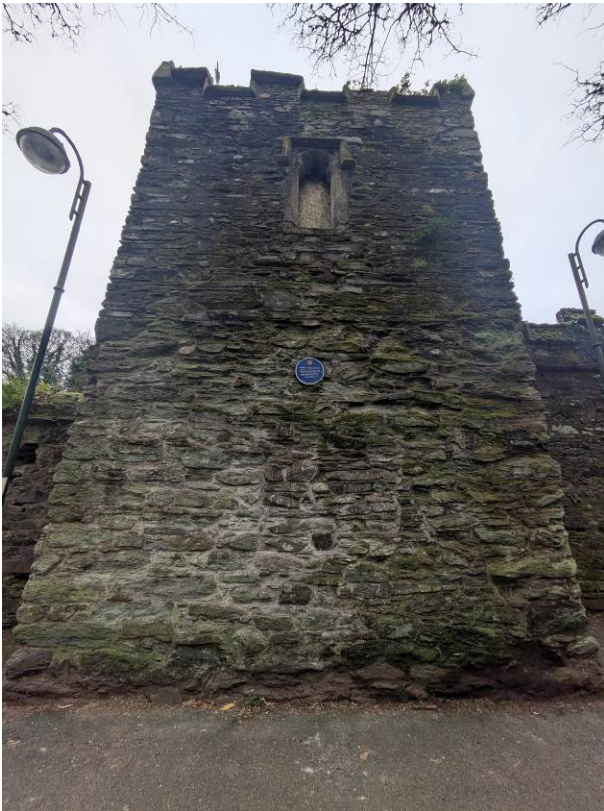
South Elevation with a large amount of Damp Stonework ( Image 5 )
