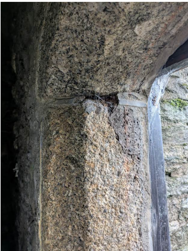
Failed Inappropriate Cement Pointing to Upper Storey Granite Door Surround ( Image 15 )
