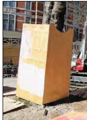
Figure 2.03– Example of final tree trunk protection measures.
