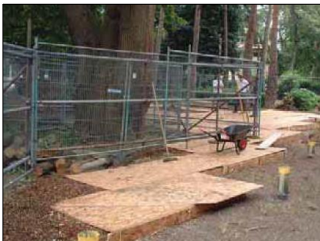
Figure 2.05 – Example of ground spreader boards atop of a compressible layer of woodchip for use on this Site.
