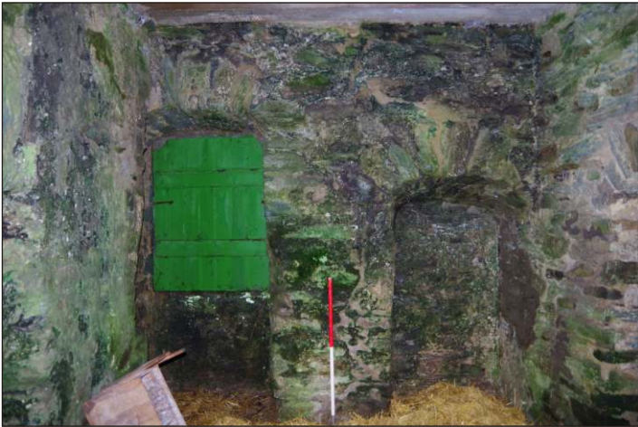
Plate 32: Ground-floor east elevation of the Still House, looking northeast. (1m scale)
