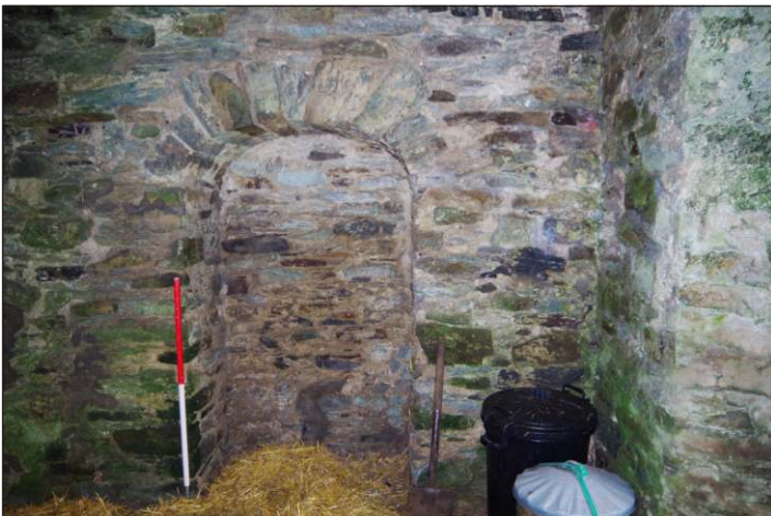
Plate 33: Ground-floor south elevation of the Still House, looking east-southeast. (1m scale)
