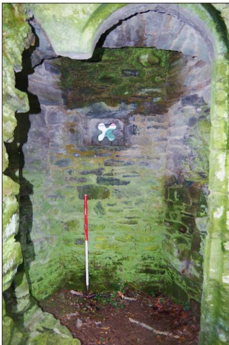
Plate 15: Ground-floor Garderobe in north turret of Betsy Grimal's Tower looking west-southwest. (1m scale)
