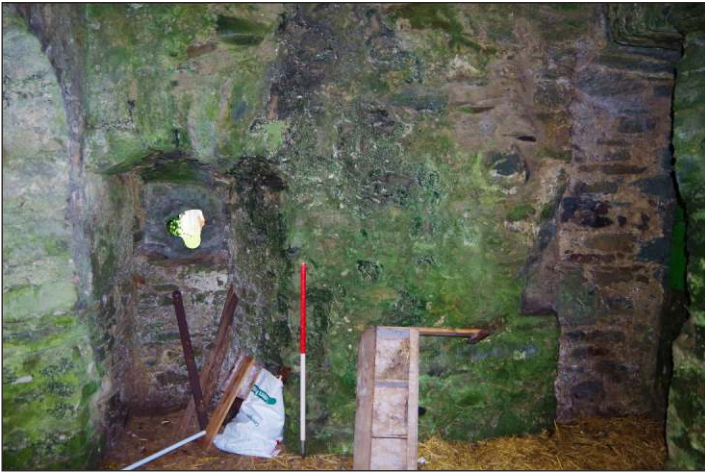
Plate 31: Ground-floor north elevation of the Still House, looking northwest. (1m scale)
