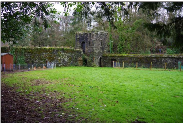
Plate 25: Location shot of the Still House, looking southeast. (1m scale)
