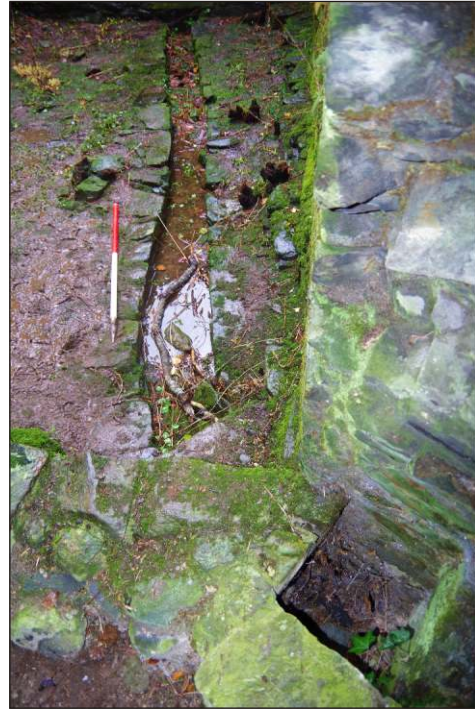
Plate 14: Drain in north wing and garderobe drain of Betsy Grimal's Tower, looking northeast. (1m scale)
