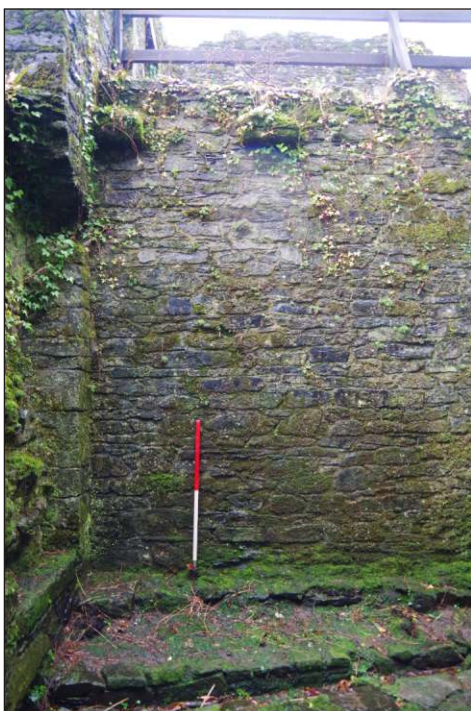
Plate 12: South elevation of north wing of Betsy Grimal's Tower, looking east-southeast. (1m scale)
