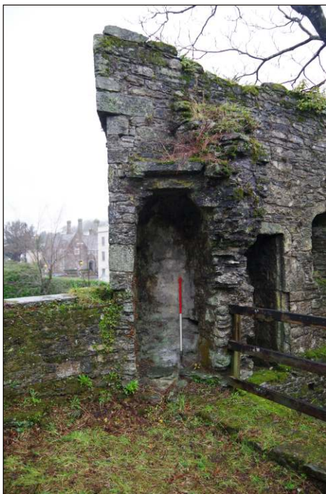
Plate 23: First-floor garderobe and stub of north elevation of Betsy Grimal's Tower, looking west. (1m scale)
