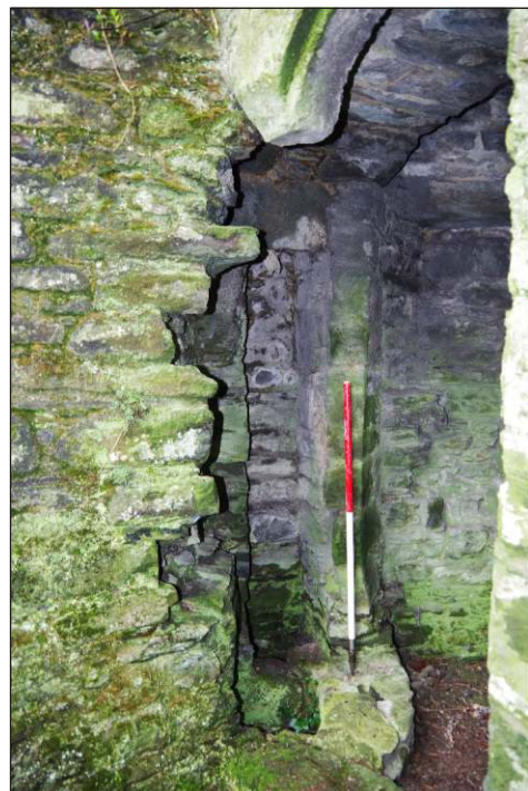
Plate 16: Exposed drain of first-floor Garderobe in ground floor garderobe of Betsy Grimal's Tower. (1m scale)
