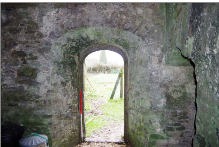
Plate 34: Ground-floor west elevation of the Still House, looking southeast. (1m scale)
