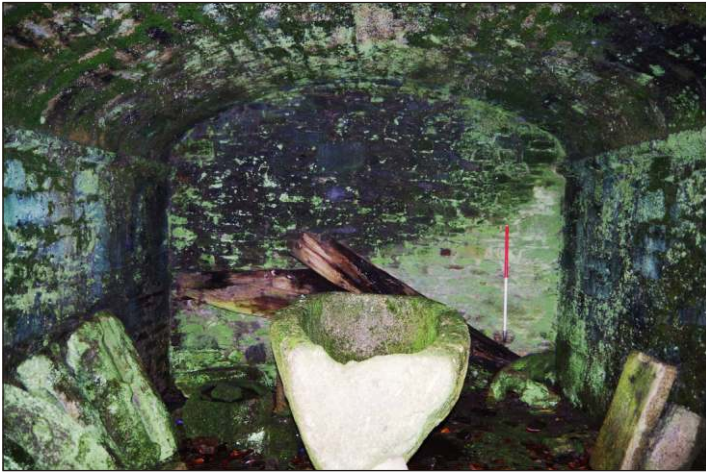
Plate 8: East end of the gate-hall of Betsy Grimbal's Tower, looking east-northeast. (1m scale)
