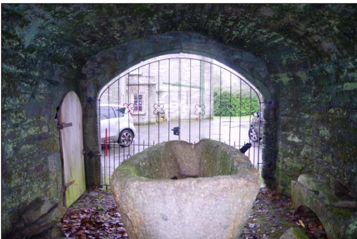
Plate 9: West end of the gate-hall of Betsy Grimbal's Tower, looking west-southwest. (1m scale)
